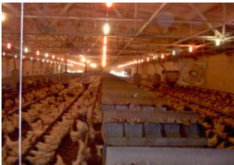
Pic. 2. Laying nests placed across the direction of airflow will limit the efficiency of tunnel ventilation'
